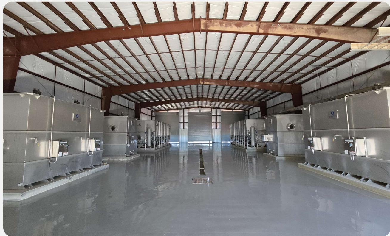
Auxiliary Facility Construction
