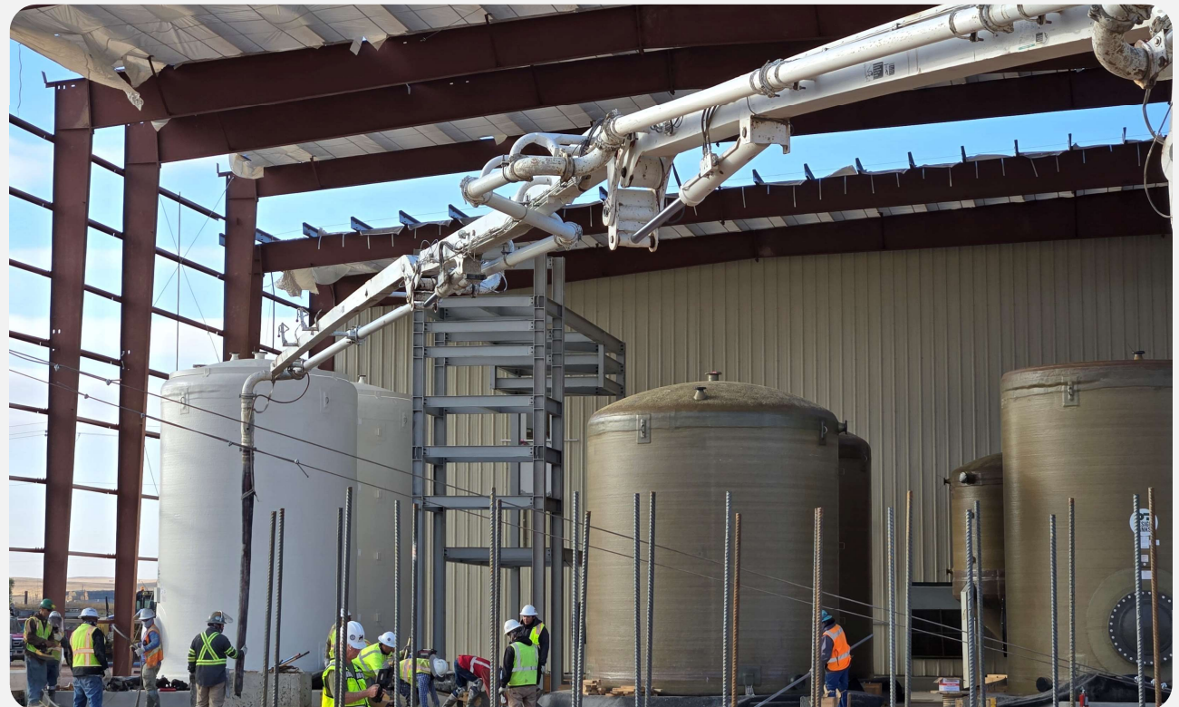
Pouring plant concrete and setting tanks
