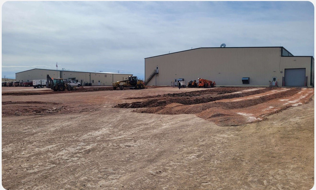
Early Earthworks in advance of Construction
