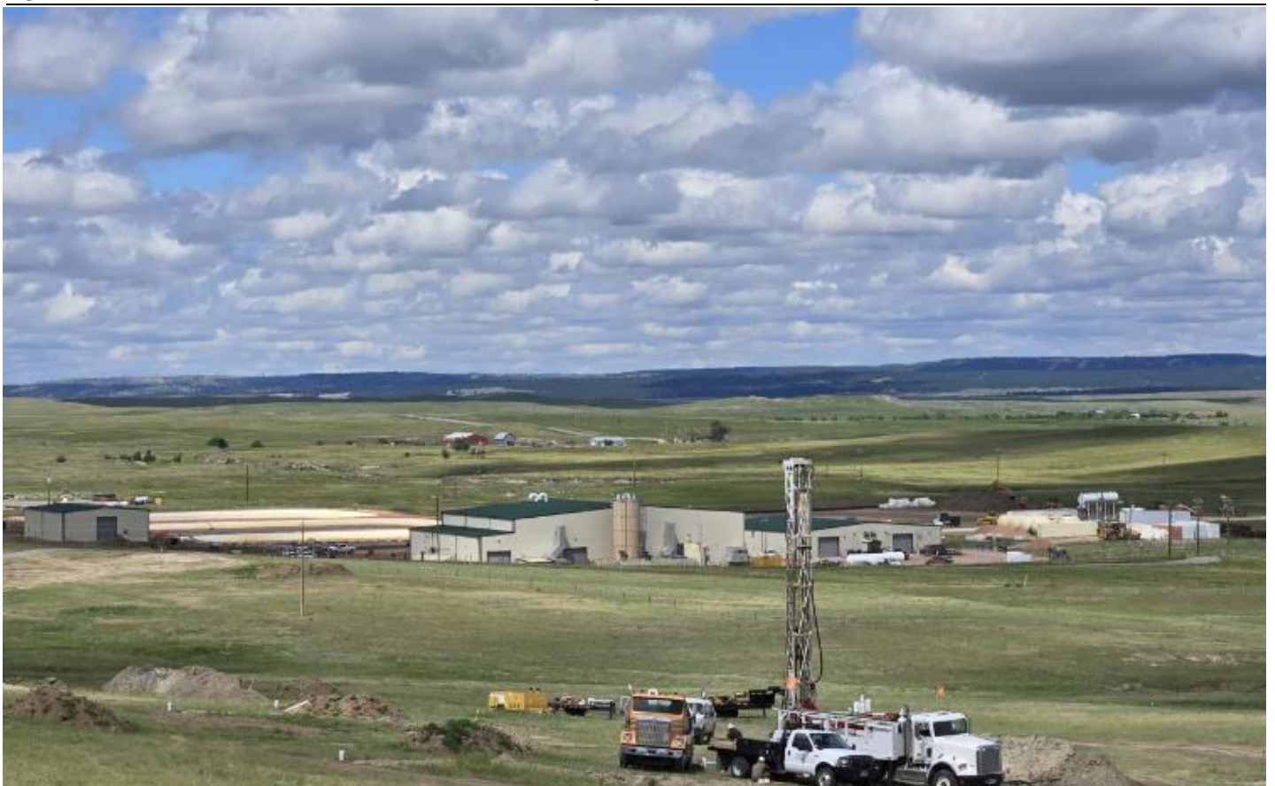
Figure 4: Active well installation at Mine Unit 3. Ross Plant in background.
