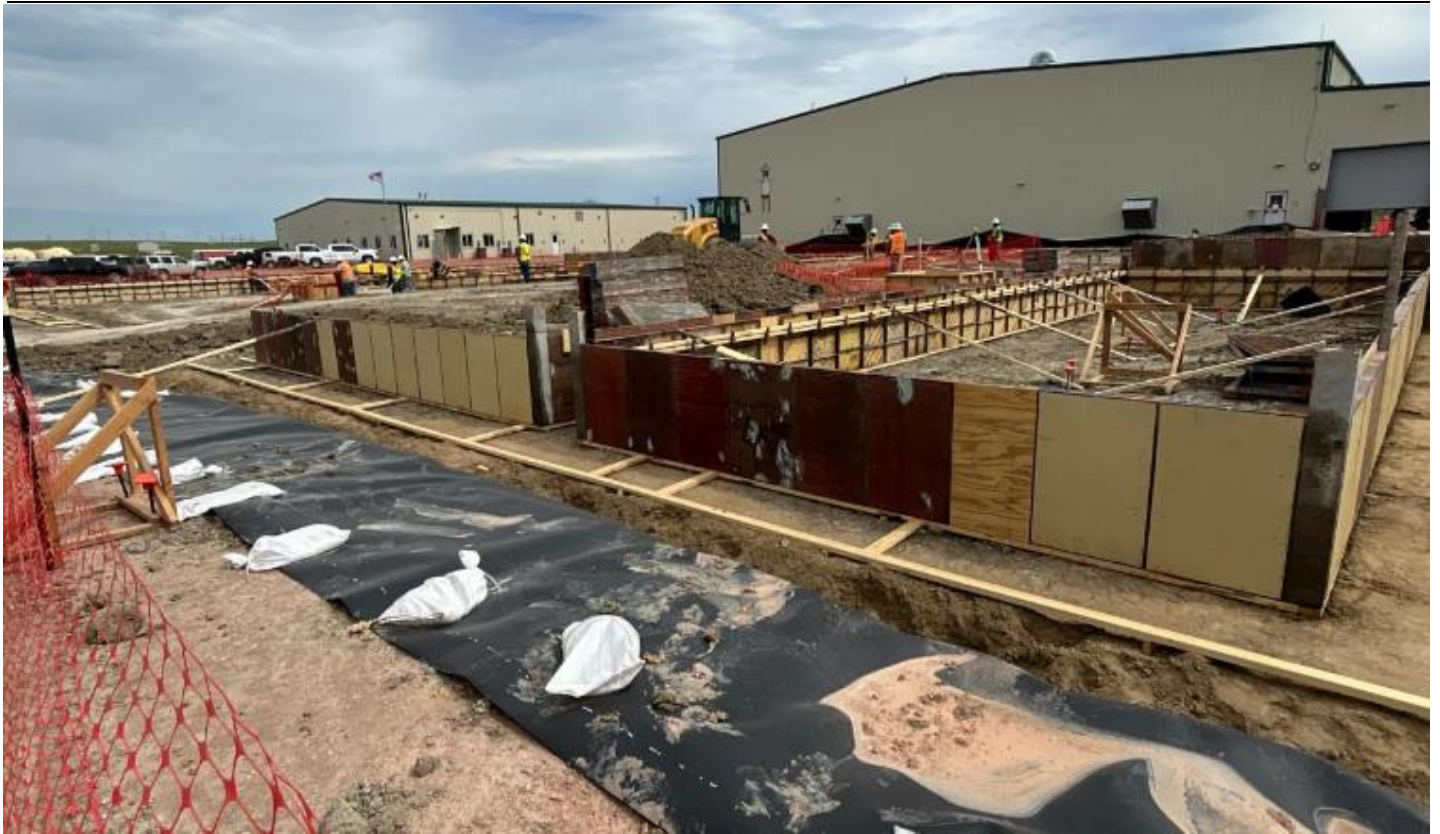
Figure 3: Crews installing forms in preparation for upcoming concrete pours at Ross CPP site
